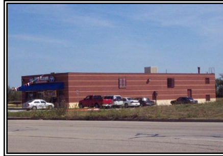
Lack of Articulation: Even extensive treatment of landscaping, awnings, and other frills cannot overcome a structure that has no variety in its horizontal and vertical surfaces
