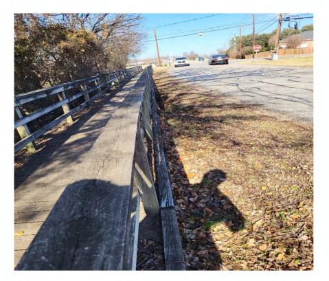
Some maintenance is required screws to be added, boards replaced, power washed, and
